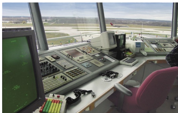
A view of the inside of the Air Traffic Control Tower cab at GFIA.
