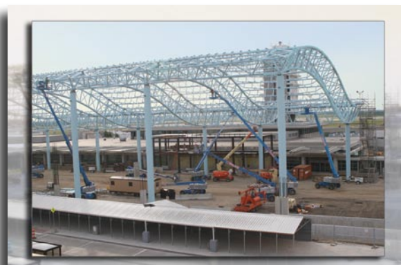
The first six girders are up. The temporary terminal curb front can be seen in the foreground. (Photo taken from the fourth level of the parking deck.)
