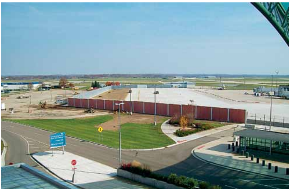
The new Concourse B ramp project as seen from the east end of the parking garage.
